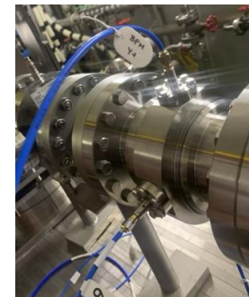
Figure: CEA Saclay cBPM installed at ATF
