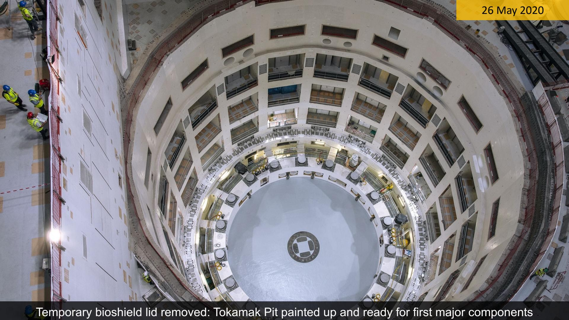
Temporary bioshield lid removed: Tokamak Pit painted up and ready for first major components
