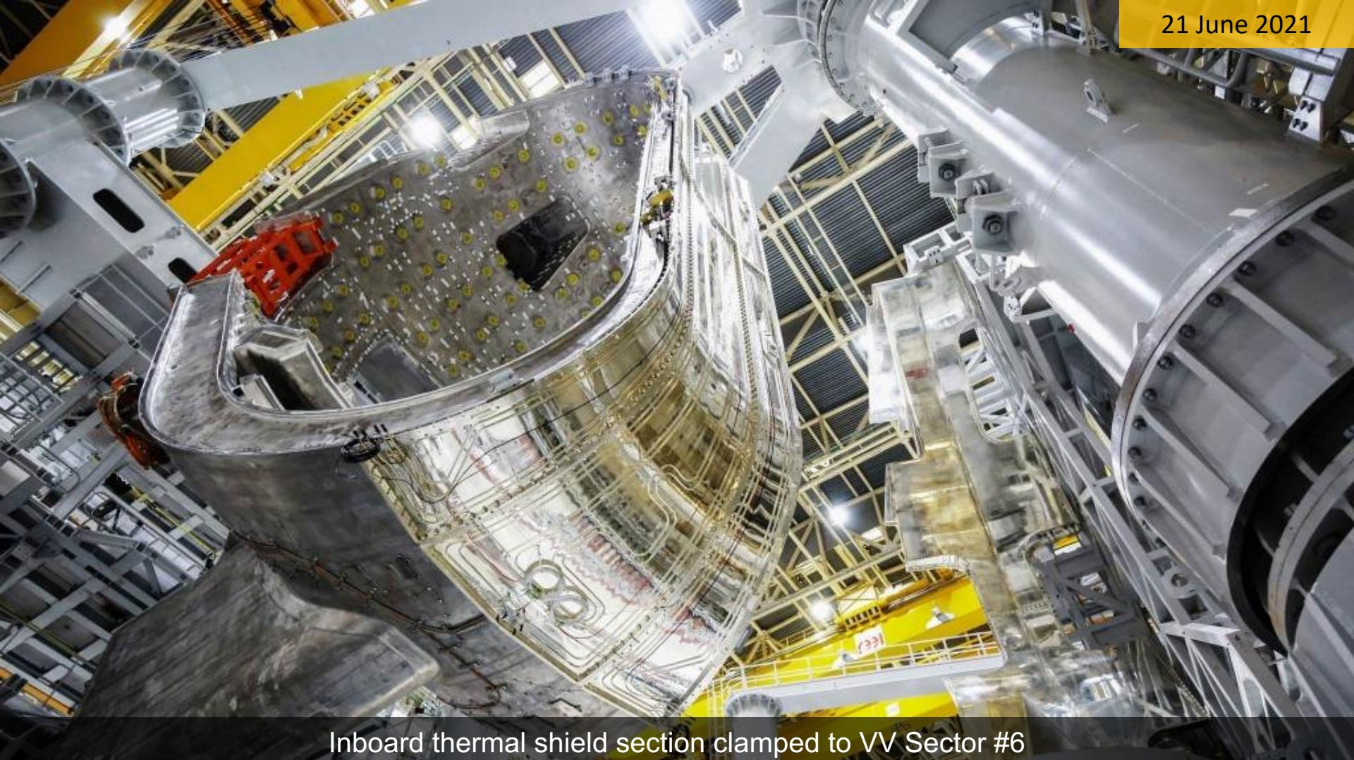
Inboard thermal shield section clamped to VV Sector #6
