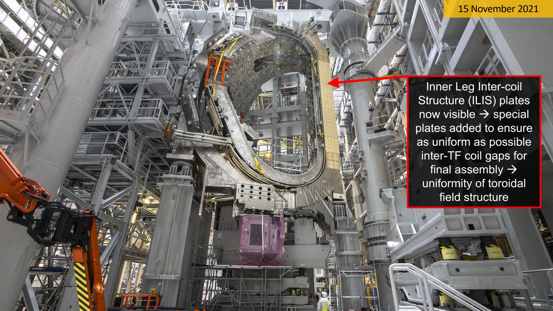
Inner Leg Inter-coil Structure (ILIS) plates now visible → special plates added to ensure as uniform as possible inter-TF coil gaps for final assembly → uniformity of toroidal field structure
