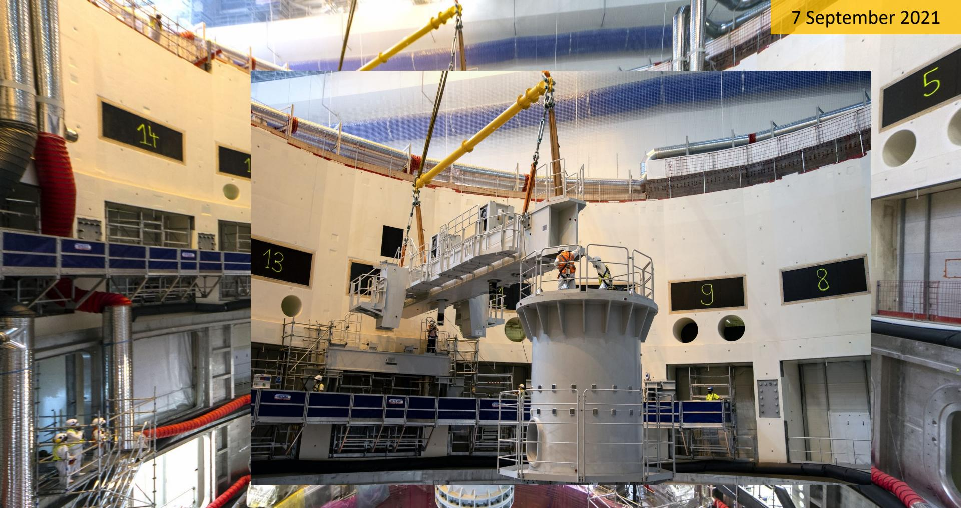
Radial beam testing → beams carry each VV sector and must be very precisely positioned
