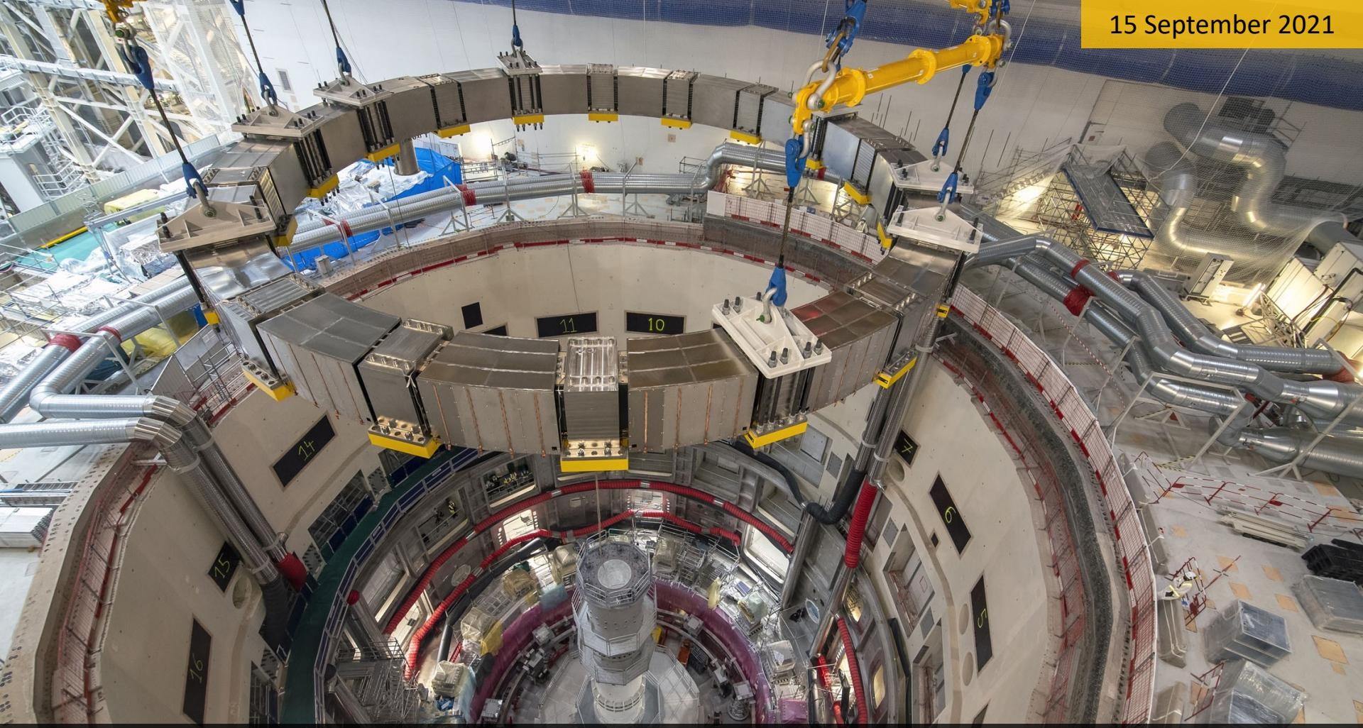
PF 5 coil lifted into the tokamak pit
