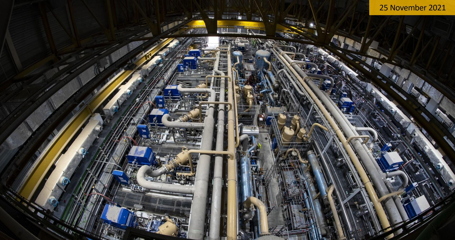
Over 5000 t of equipment installed in the cryoplant in 3.5 years → 2 year commissioning period started
