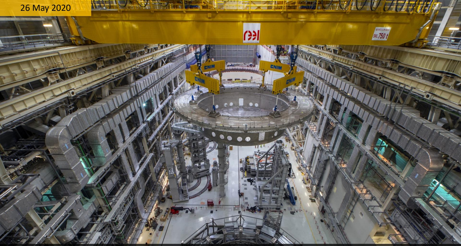
The big lift: 1250 tonne, 30 m diameter cryostat base on its way to the pit
