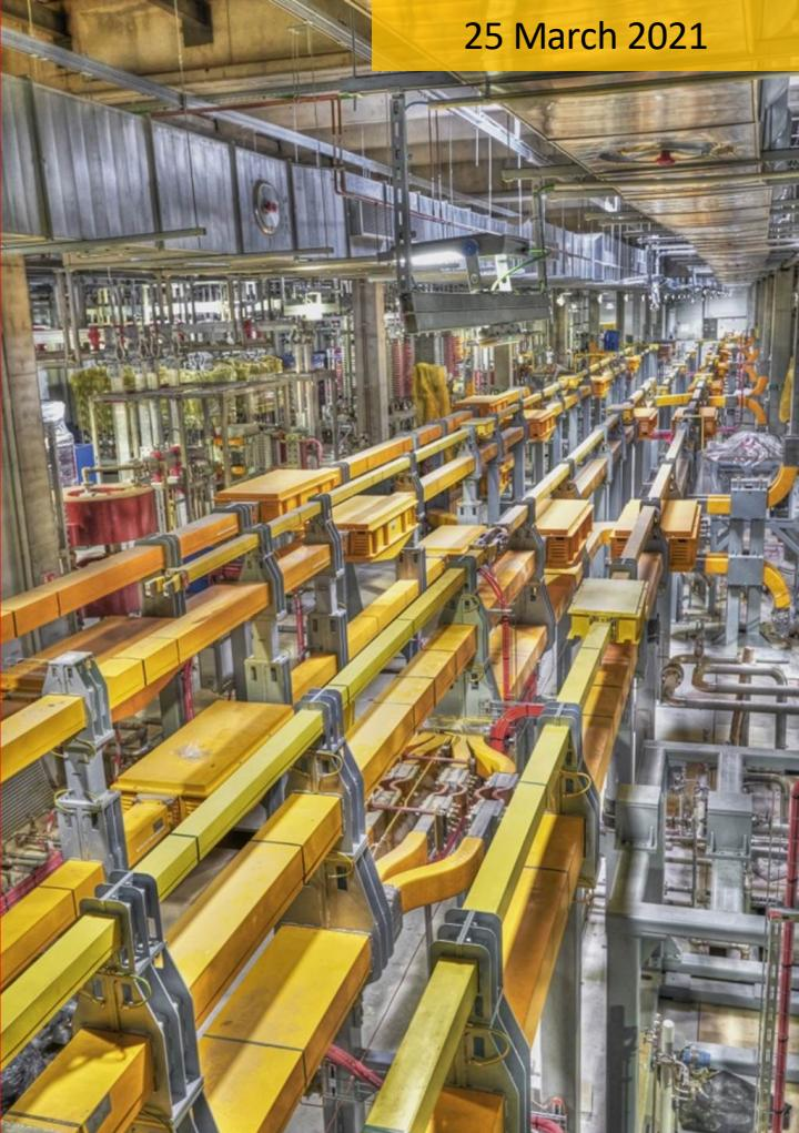
Magnet conversion buildings filling up with DC busbars for superconducting coils
