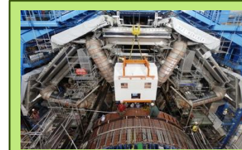
SCT+TRT Barrel Installed with in ATLAS August-2006
