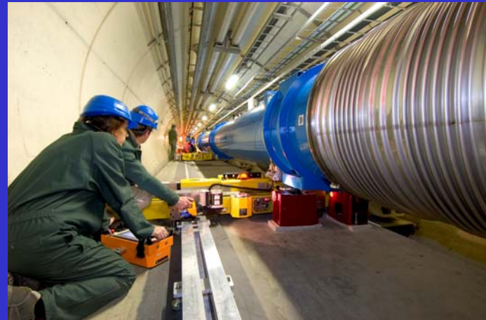
Installation work, underground
